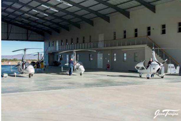
In the massive hangar at Karoo Gateway
