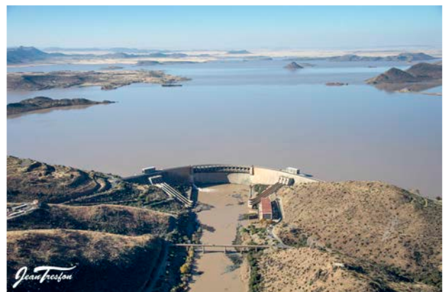
Flying over the Gariep Dam wall
